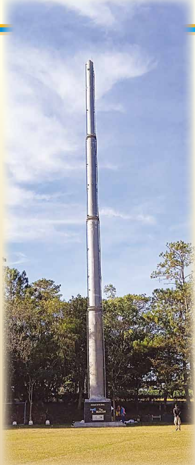
Full view of the Beacon from 60 meters.
