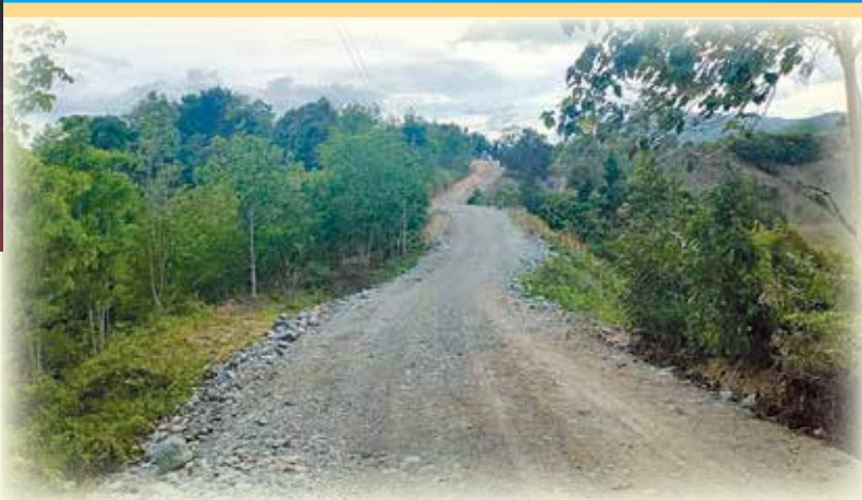
Completed 6-km Road Opening from Brgy Datu Tutukan to Labangon, Dumingag, ZDS.
