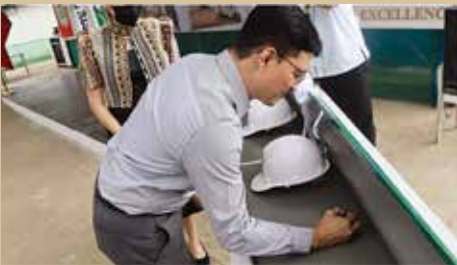
DND Undersecretary for Civil, Veterans and Reserve Affairs signs the last roof flashing.
