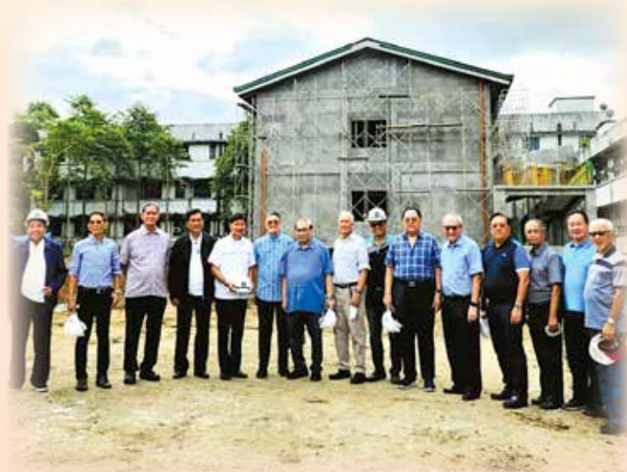
M70WW as work-in-progress 2023.
