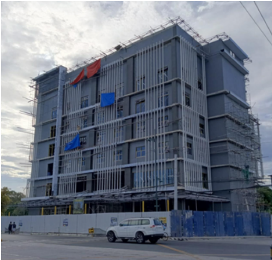
Current state of the PMAAAI Building
